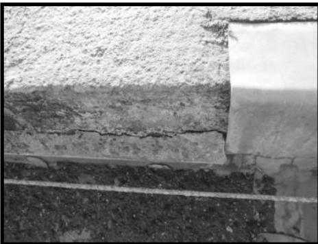
Fig 2: Cracking at the joints between the stone, lead flashings and the lime-mortar infill.
