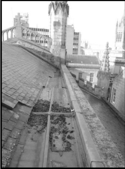
Fig 1: Moss and debris accumulation in the valley gutters. Looking towards the west gable on the nave roof.
